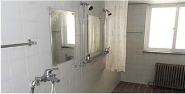
Building No. 3 shower stalls
