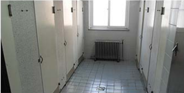
Building No. 3 bathroom
