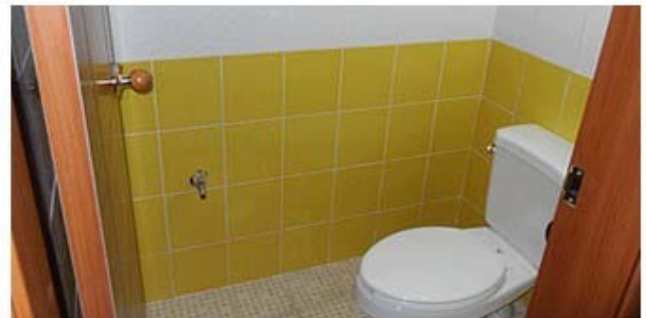
Building No. 4 bathroom
