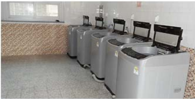
Building No. 4 laundry room
