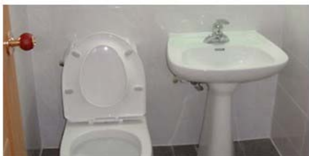
Building No. 5~6 bathroom
