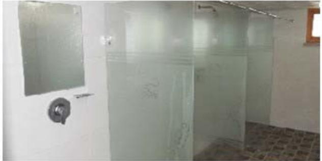
Building No. 1 shower stalls
