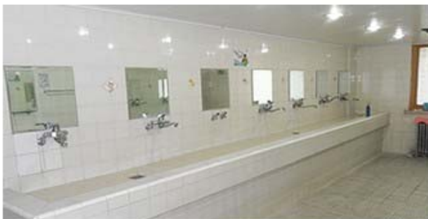
Building No. 1 washroom
