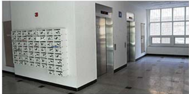
Building No. 4 lobby
